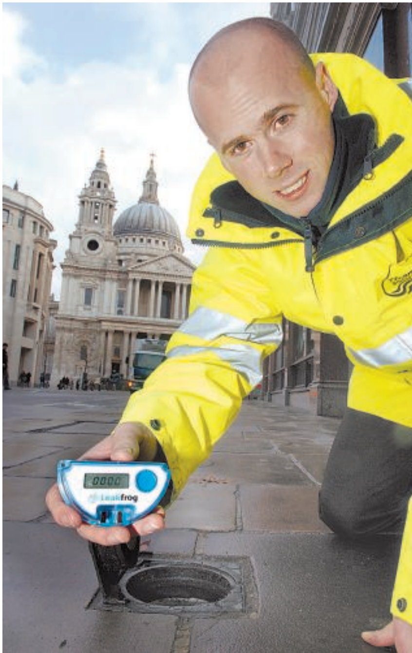
Thames Water installs a Leakfrog on a meter outside St Paul's cathedral
